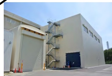
COMET & Control room
